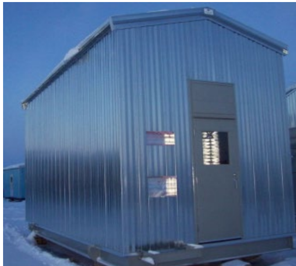
Example Dosing Building
