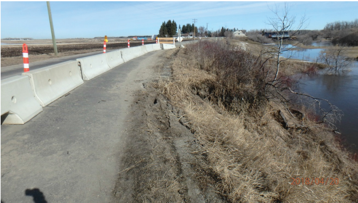
Photo 4 Portions of the slope with a north facing aspect were still covered with snow at the time of KCB's site visit. Note highwater in Sturgeon River that precluded inspection of the toe of the slope at normal water level. Photo taken on April 20, 2018 looking south east.
