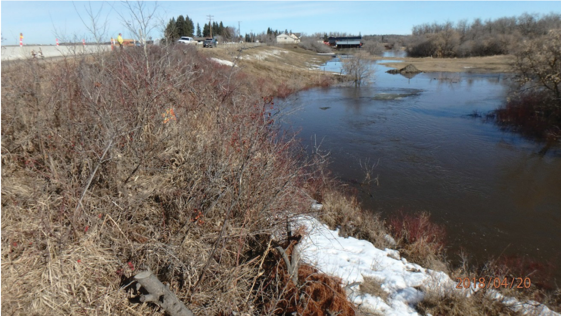
Photo 6 A portion of the slope to the north of the active failure zone is in the process of failing, and will enlarge the slide area. Red arrow shows location of ground cracking associated with expansion of slope failure area. Photo taken on April 20, 2018 looking north.
