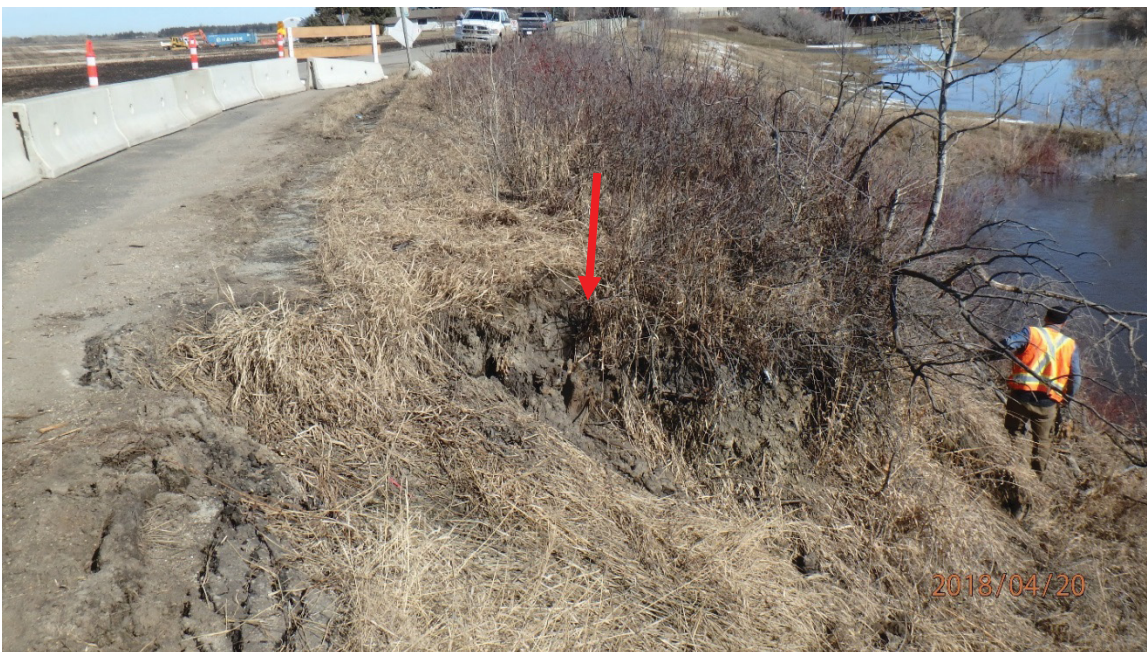
Photo 6 A portion of the slope to the north of the active failure zone is in the process of failing, and will enlarge the slide area. Red arrow shows location of ground cracking associated with expansion of slope failure area. Photo taken on April 20, 2018 looking north.
