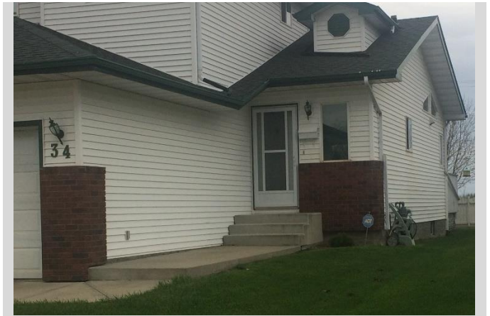
Image 2.2 Downspout House 34 (Not connected to sanitary system)
