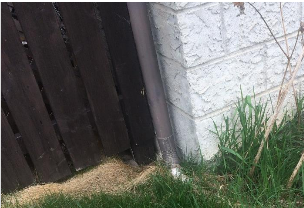
Image 2.7 Downspout House 83 (Not connected to sanitary system)
